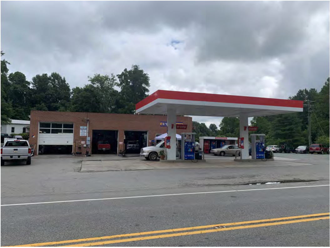
EXISTING - TAKEN FROM ACROSS RT. 250
