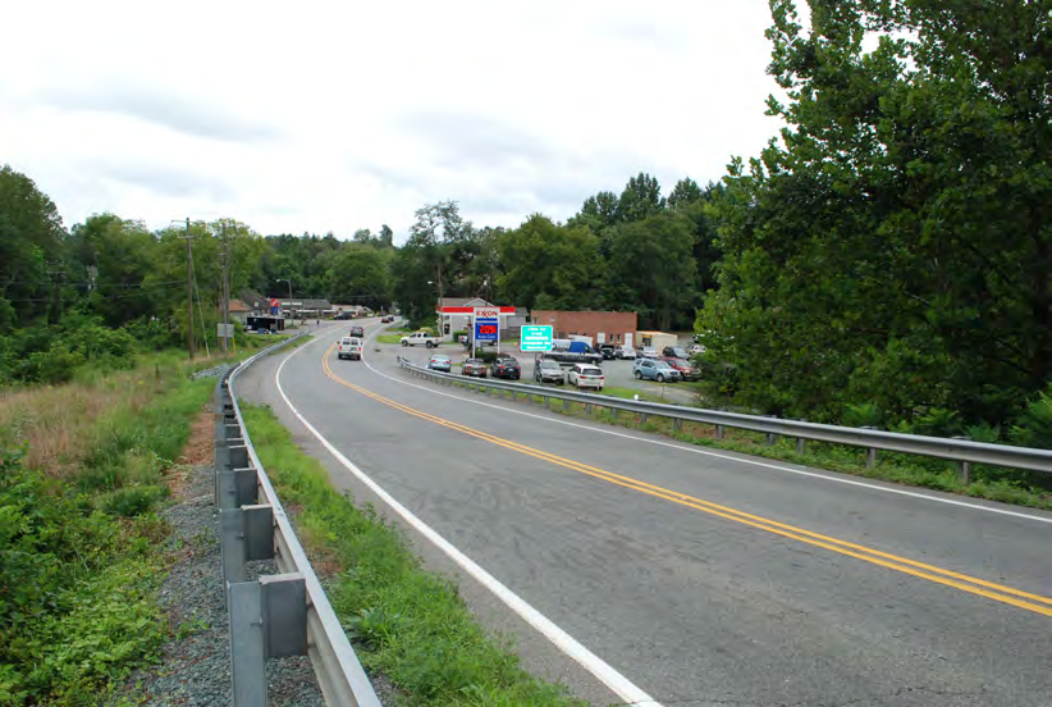
EXISTING APPROACH FROM RT. 250 HEADING WEST
